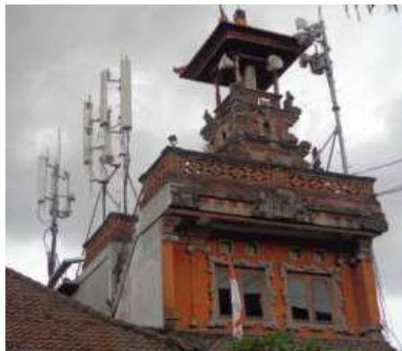
Fig. 3 Rooftop tower at banjar hall
