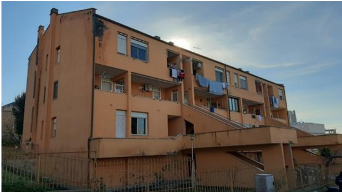
Fig. 6. ATER building north-west view
