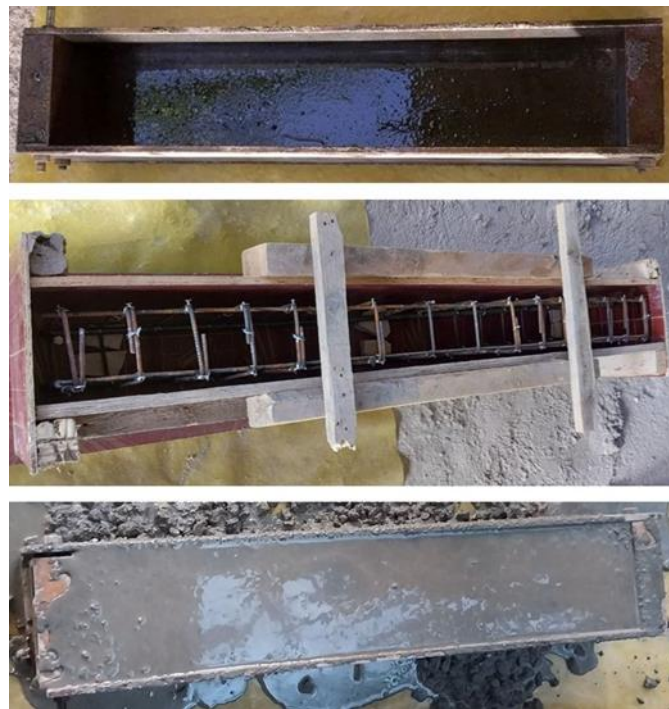
Figure 3. Steps of making laboratory samples of reinforced concrete beam.
