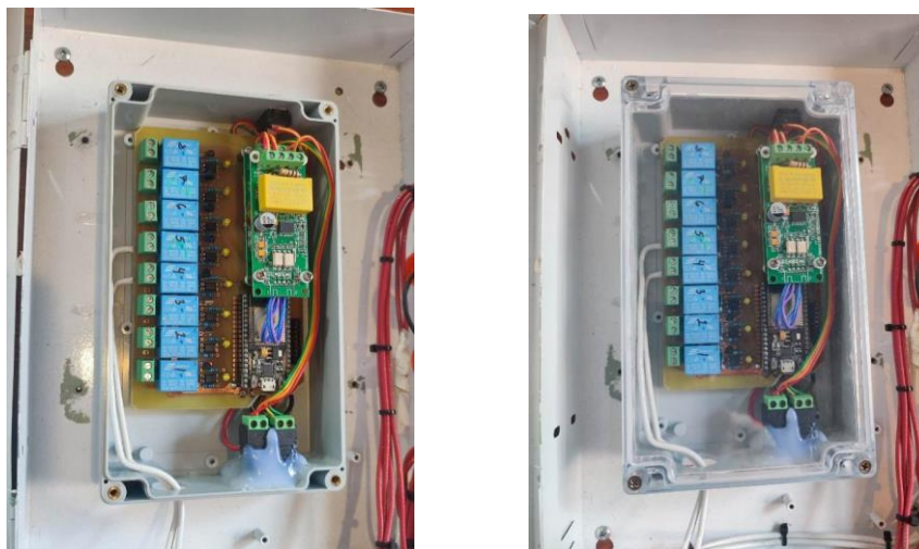
Figure 4. IoT Home Automated and Technology-Based Smart Energy Metering System with Data Analytics
