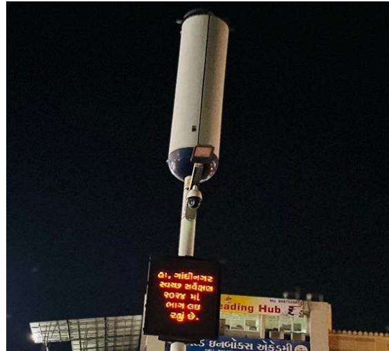
Figure 9. Existing System – Sector 6, Gandhinagar, Gujarat
