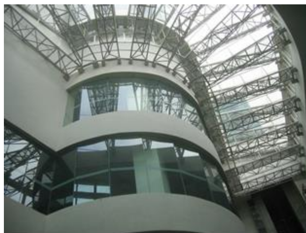
Figure 4.1 Vertical glass glazing is present on a two-
