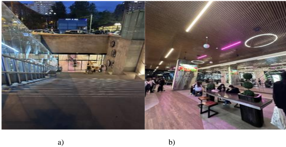
Fig. 3. a, b - "No. 1" underground area built at the intersection of Mashtots and Aram streets in Yerevan 4
