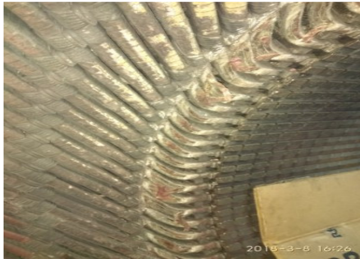
Fig. 7. Deformation of 15 MW, alternator due to dislocation.
