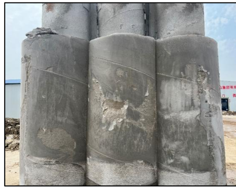
(b) Photo of grouting compaction specimen
