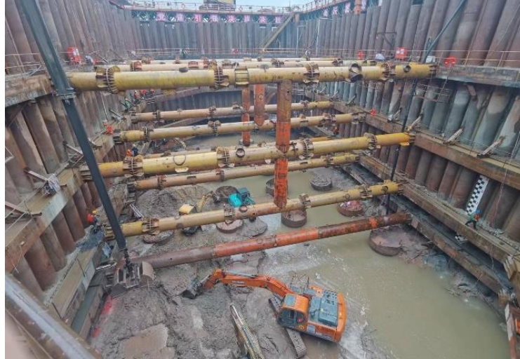
Figure 9: Photos of On-site Foundation Pit Excavation
