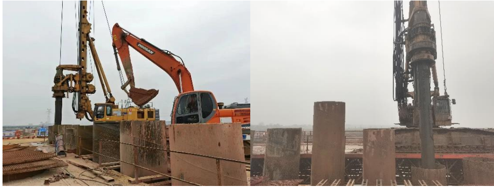
Figure 7: Photos of On-site Rotary Drilling Pilot Hole Construction
