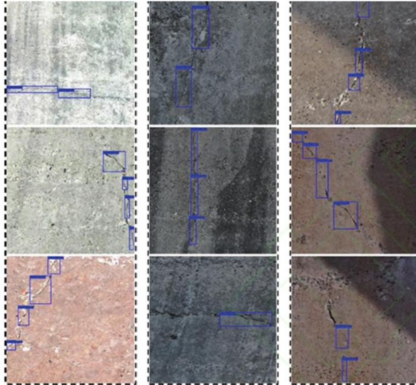
Fig.7 Crack image detection results under different lighting environments
