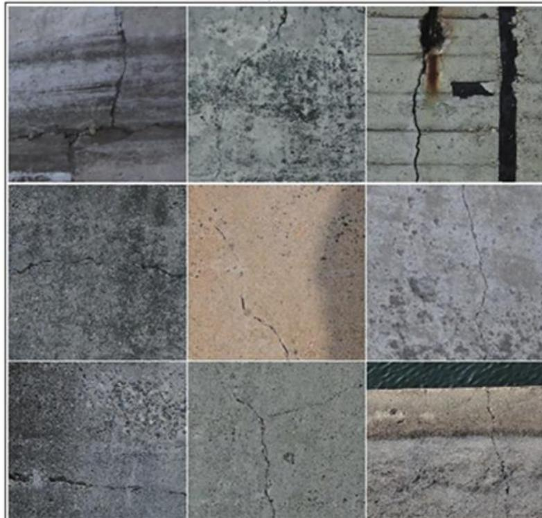
Fig. 3 Example of crack image acquisition for concrete dam
