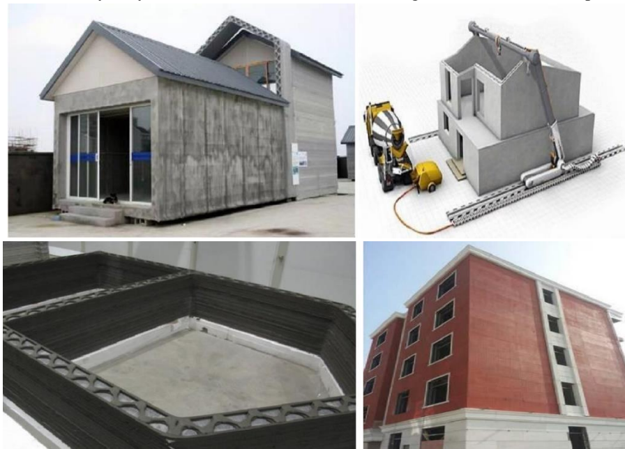
Figure 12: 3D Printing Buildings
