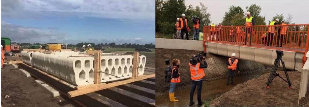
Figure 13: 3D Printing Bridges
