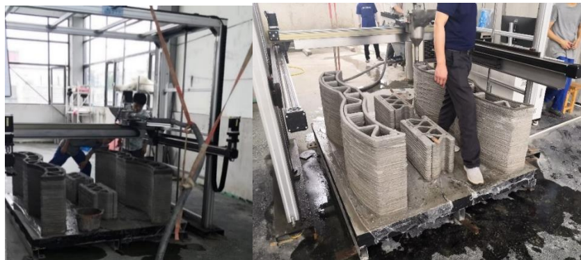
Figure 11: Field application of Concrete 3D Printing Formwork
